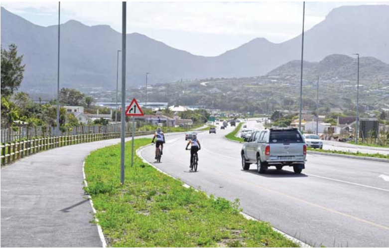
Room to ride: The mammoth R194 million project to relieve traffic congestion on Kommetjie Road, which started in October 2016, is now complete.
